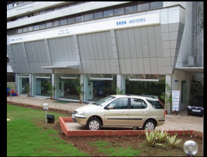
Project : Fortune Cars Pvt. Ltd. Type of Work : Show Room Quantum of Work : 2,000 Sft.
