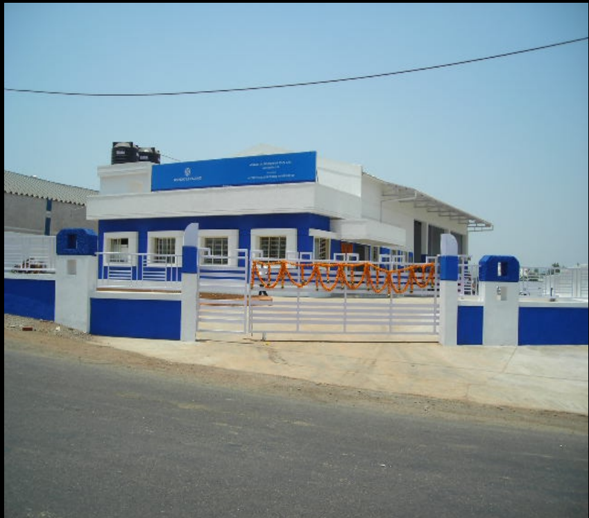
Project : Avsar Automotive Pvt. Ltd., Type of Work : Factory Building Quantum of Work : 50,000 Sft.
