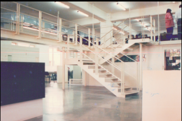
Project : B.J. Medical College Type of Work : Library Quantum of Work : 10,000 Sft.
