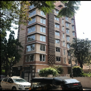
Project: Meher, Bandra West, Type of Work : Residential Building (Double Basement, Ground + Eight Floors) Quantum of Work : 28,000 Sft.
