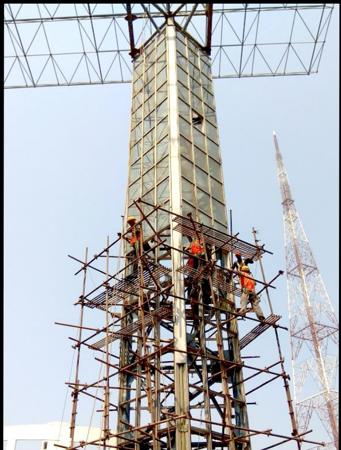
Project: Mahindra Tower, Worli Type of Work : 90 feet column repair
